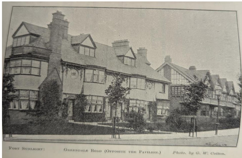
Figure 9: Greendale Road (Opposite the Pavilion). Port Sunlight Monthly Journal , February 1897, Vol 3, No. 2, page 46.
